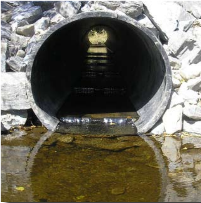
Pools adjacent to culvert can play important design elements in aquatic passage.
