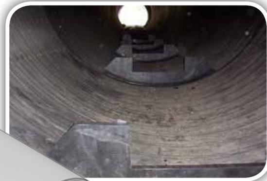
*The notched weir baffle design and corner baffle designs are recognized by the Federal Highway Administration along with many state transportation and environmental agencies.*
