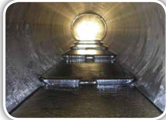
*Ponding effect created by baffle/weir design during low-flow.*
