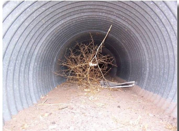
*With 8" – 10" of sediment inside the 30" CMP, the culvert had to be cleaned prior to installation of 24" Snap-Tite pipe.*
