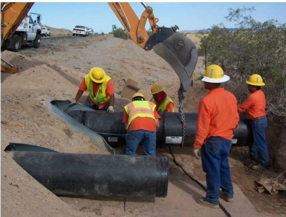
*Equipment used to align pipe.*
