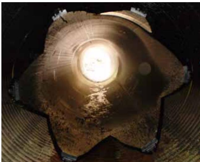
*The bullet nose Snap-Tite® end of the pipe is slid through the deflected old culvert.*
