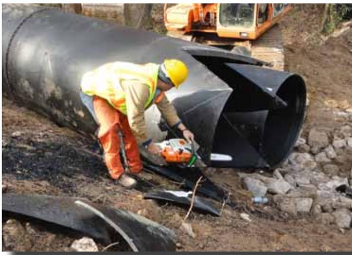
*A DOT maintenance worker cuts a bullet nose on one end of a Snap-Tite® pipe section.*
