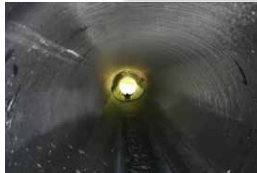
The culvert after the Snap-Tite installation.
