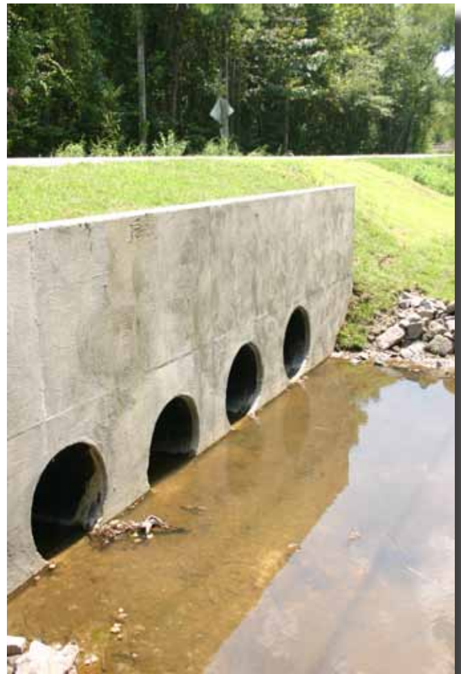
The completely rehabbed culvert.
