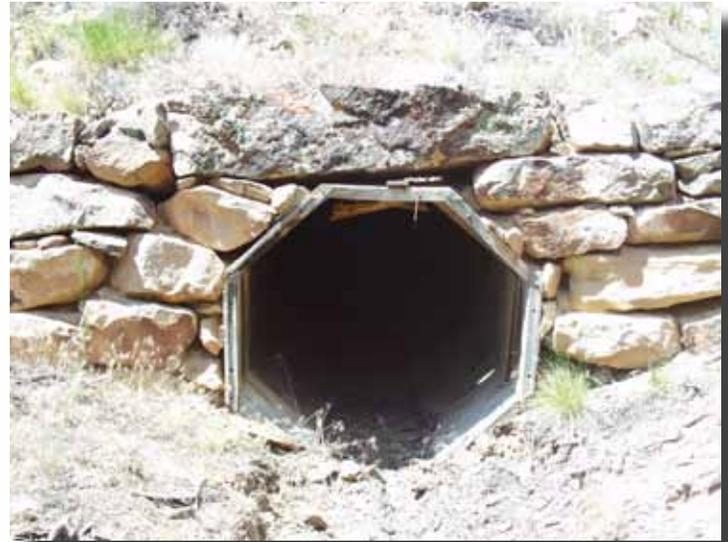
*One of the octagonal wood culverts installed in the 1920s. This one measured 36 inches in diameter.*
