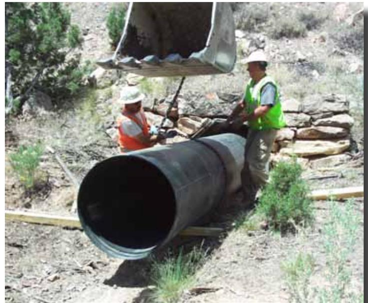
*The Snap-Tite pipe is pushed inside the old culvert. Once the snapped liner is slid in place, any annular space between the liner and culvert is filled in with grout.*
