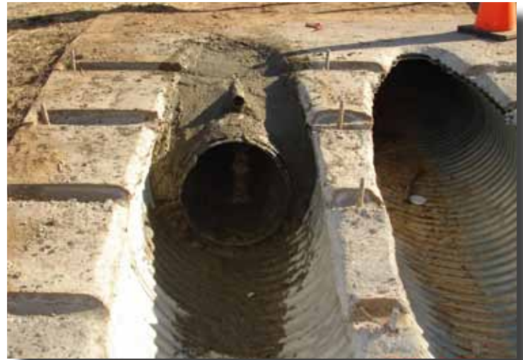
The new Snap-Tite® pipe liner installed and grouted.
