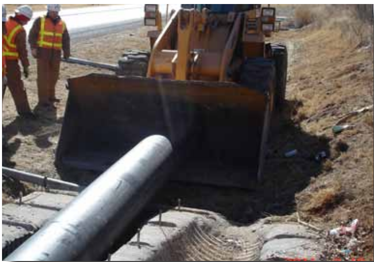
The new Snap-Tite® pipe liner installed and grouted.
