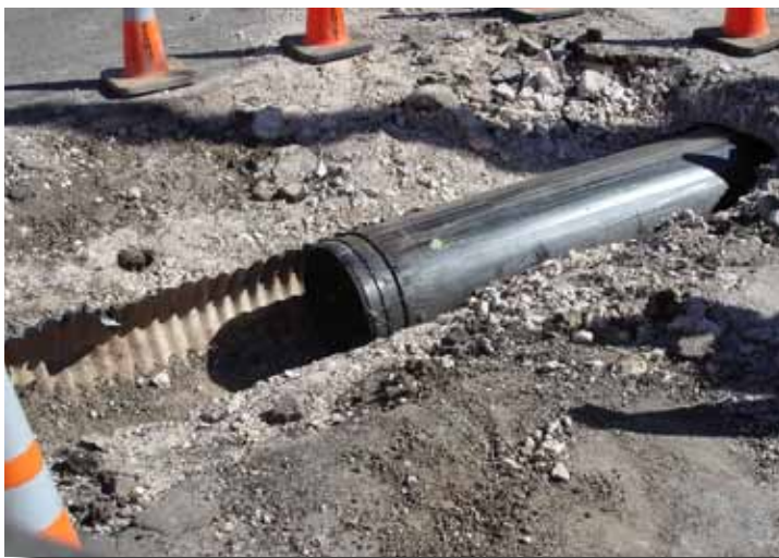
Pipe liner going in where old CMP has completely deteriorated.
