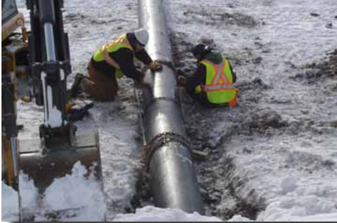
Pipe 'snapped' together at the joint and installed
