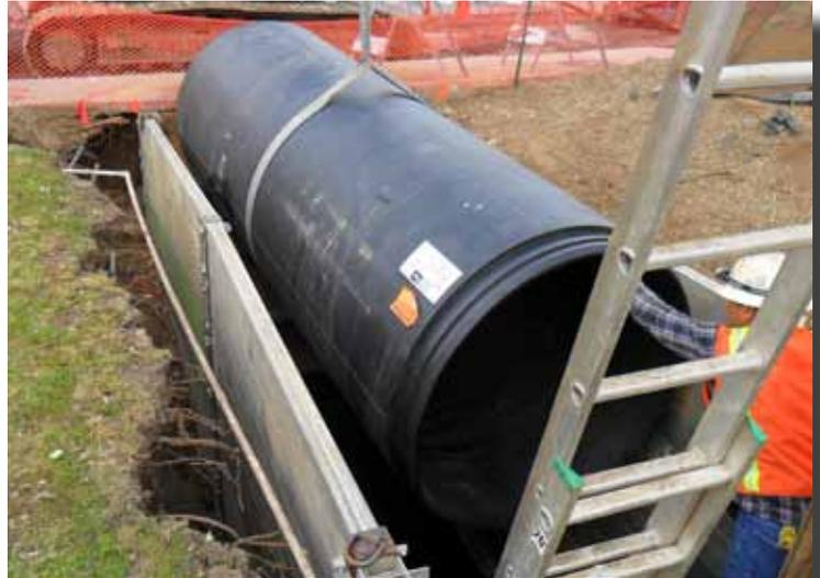
*Snap-Tite® pipe is lowered into the pit in order to reline the old CMP culvert.*
