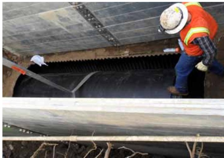
*A pipe liner section is pushed through the old existing pipe so that another Snap-Tite® section can be snapped together.*
