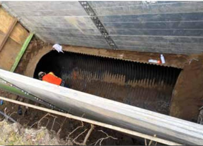
*The pit where the deteriorated culvert needed to be relined.*
