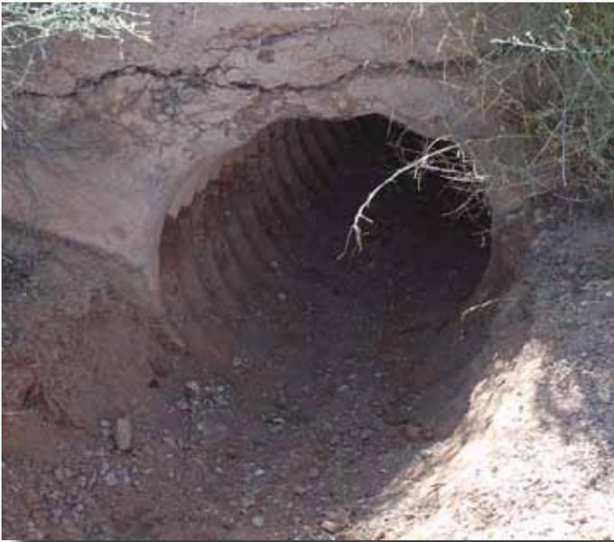
*The deteriorated corrugated metal culvert in need of repair.*
