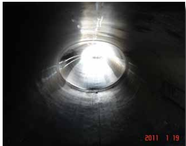
After: the culvert newly relined with Snap-Tite.
