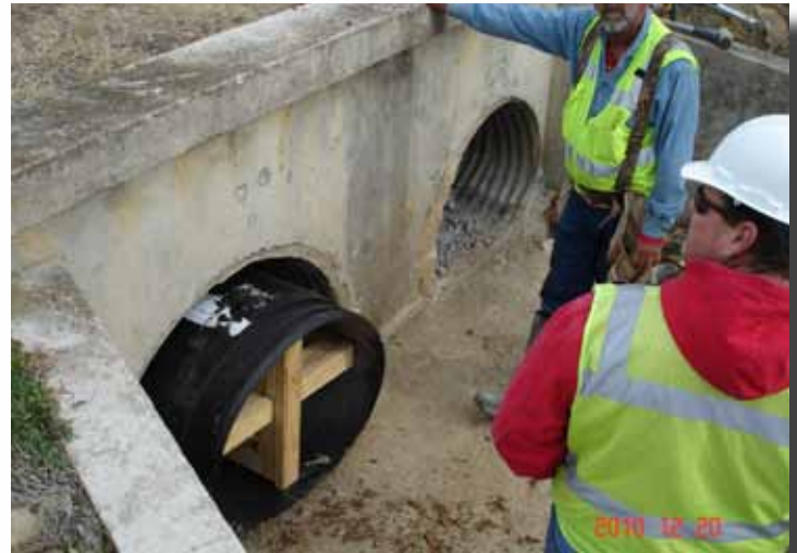
The oval-shaped Snap-Tite is slid inside the old damaged CMP.
