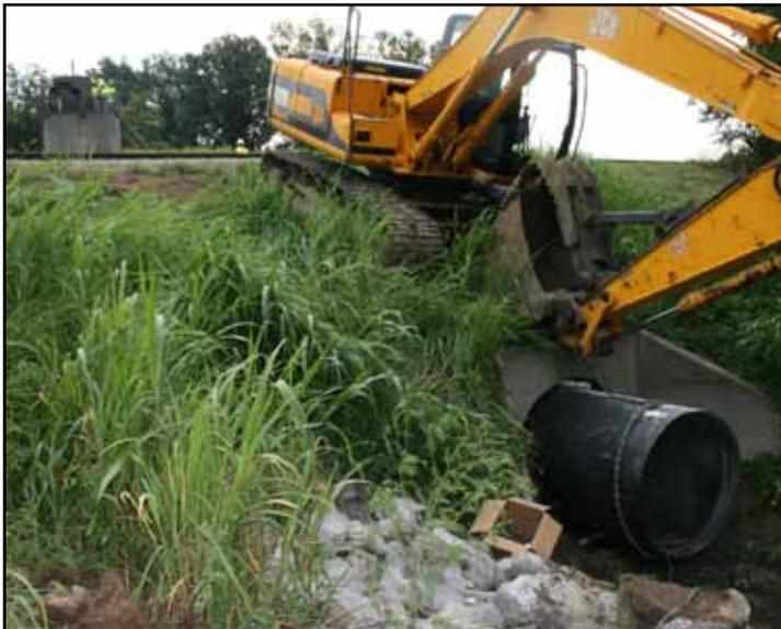
The Snap-Tite pipe was snapped together and slid inside the old levee culvert. In the background, the Hydro-Bell is being lifted into the gate house. Once inside the gate house, the Hydro-Bell was attached to the Snap-Tite pipe liner.
