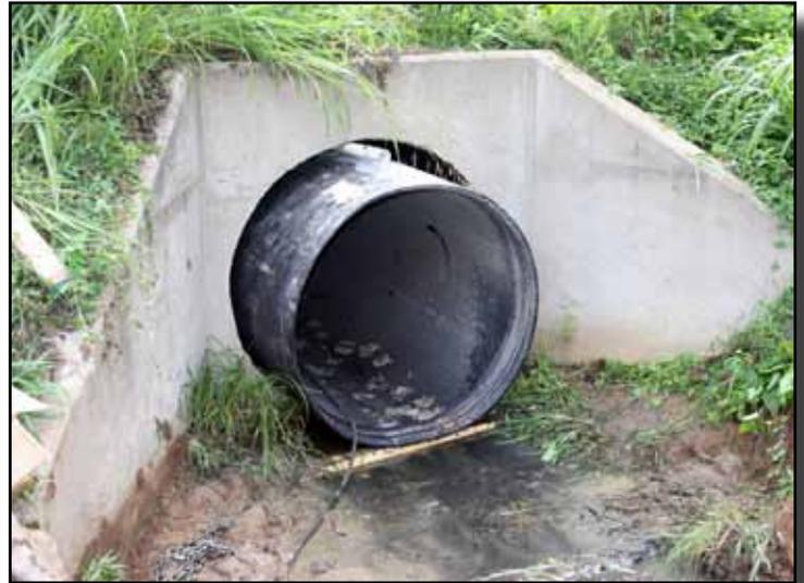
The Snap-Tite pipe is slid inside the old culvert. Once it is fully installed, grout will be used to fill in any annular space between the old culvert and new pipe.
