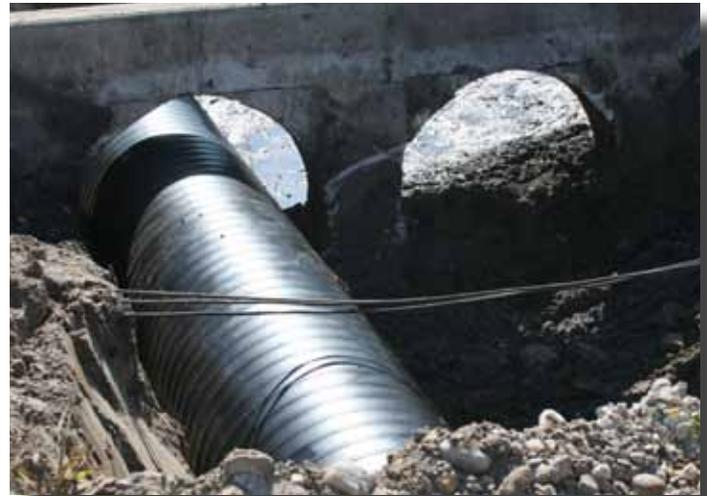
*The closed profile pipe is pushed through to reline the other damaged culvert, without having to replace the headwall.*
