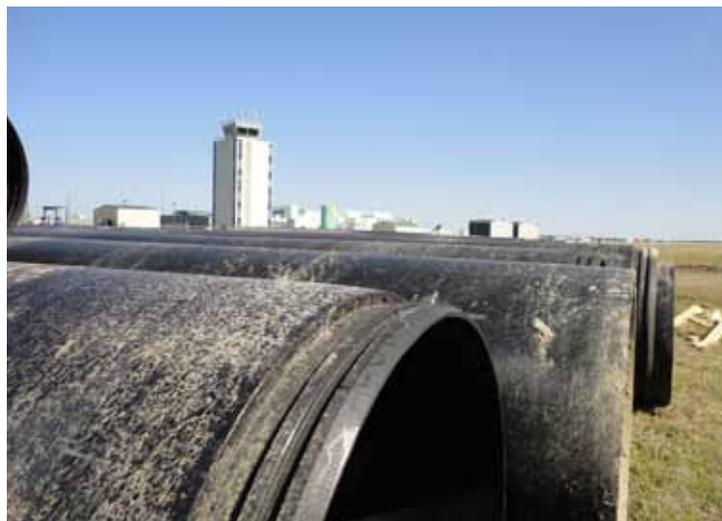
The machined ends of the Snap-Tite pipe are joined together using come-a-longs and chains. Then, they snapped sections are slid inside the old culvert.
