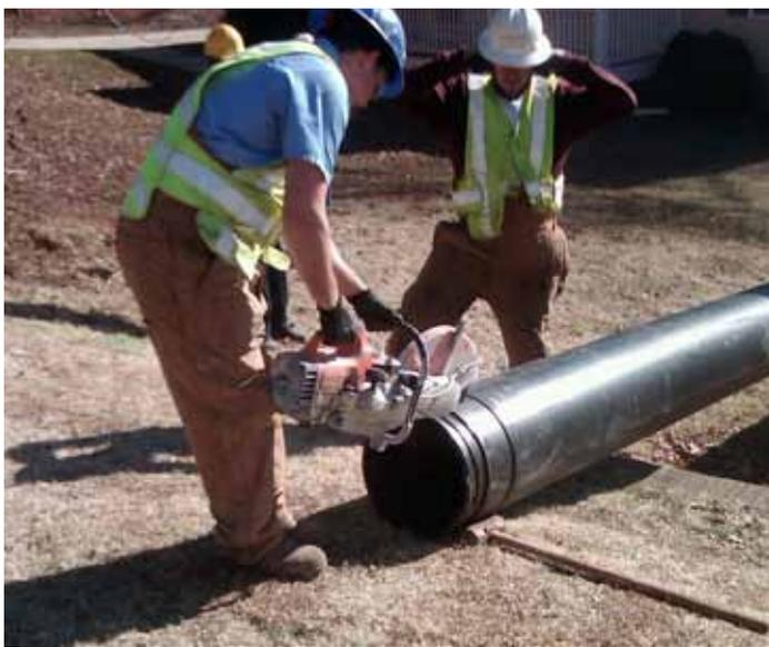
*The city's crew cuts a bullet nose into one end of the 18-inch Snap-Tite pipe liner in order to slip the liner into the deflected old CMP culvert.*
