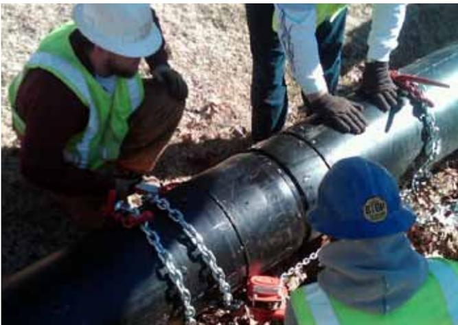
*The city's crew used come-a-longs and chains to join the sections of Snap-Tite pipe liner together before slipping the pipe into the old culvert.*
