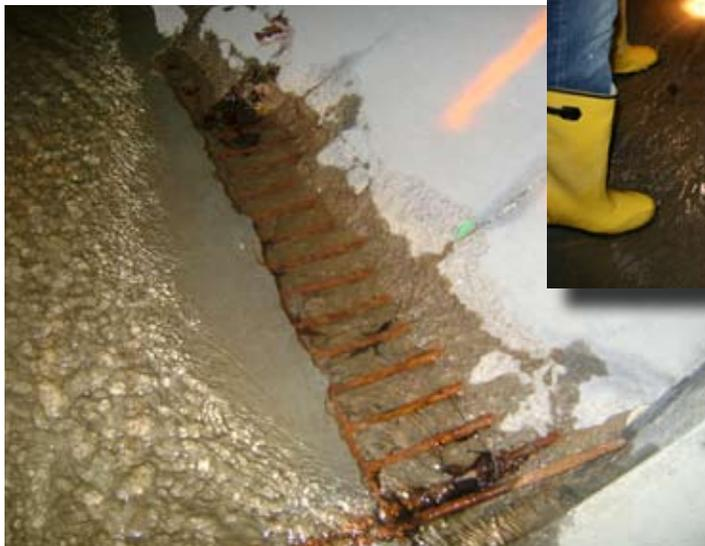
*You can see the cracking and exposed re-bar on the original RCP.*
