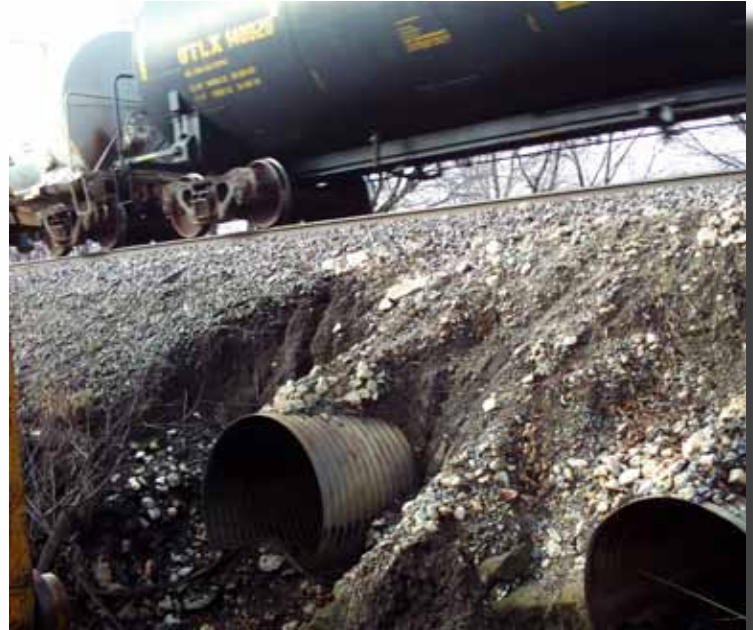
The corrugated metal pipe culverts were in bad shape and needed to be replaced without disrupting the rail service.
