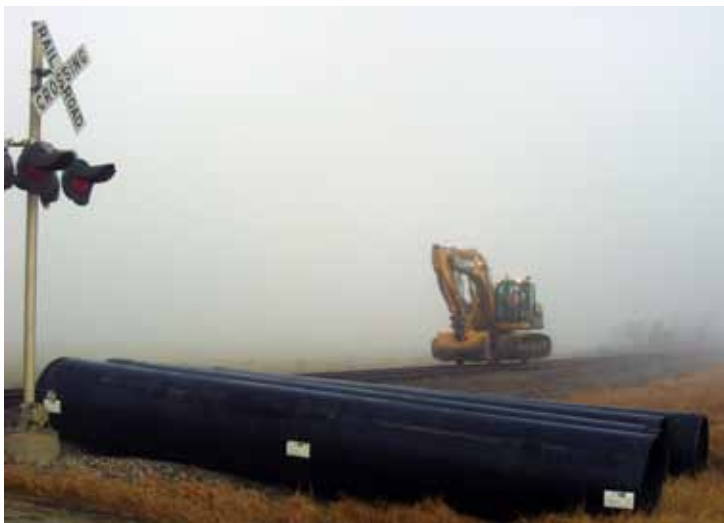
High railing the excavator to the project site. The excavator is used to push the pipe into the culvert.
