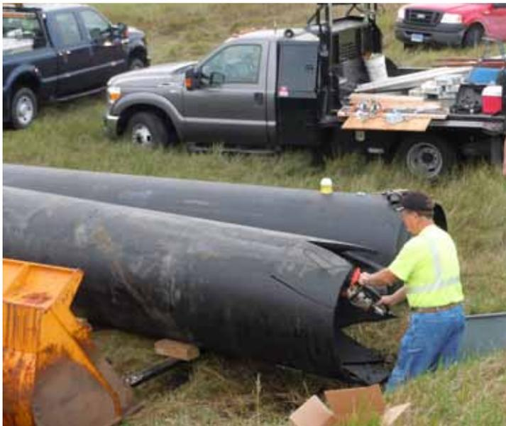
A "bullet nose" is cut on one end of the pipe liner in order to push it easily into the misshaped and damaged culvert.
