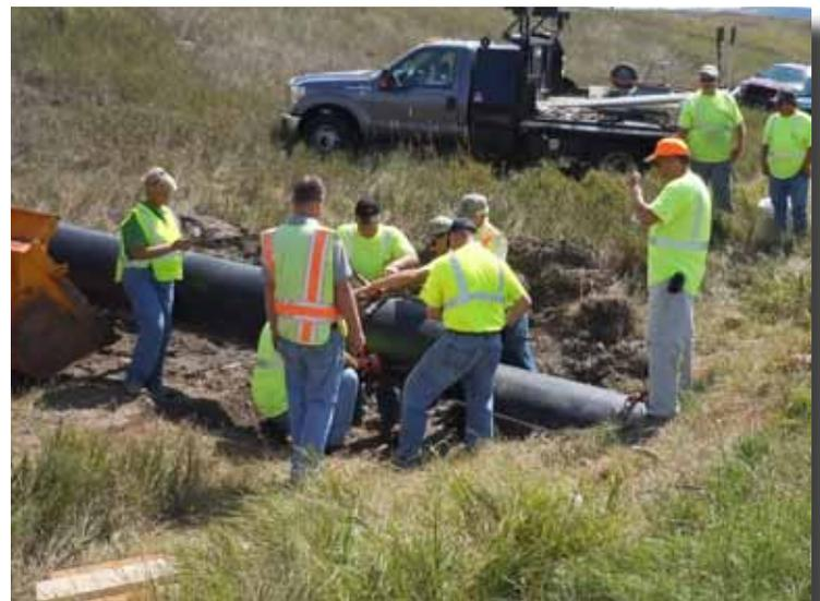
Here observers watch the lining of the 30-inch CMP with 24-inch Snap-Tite pipe.
