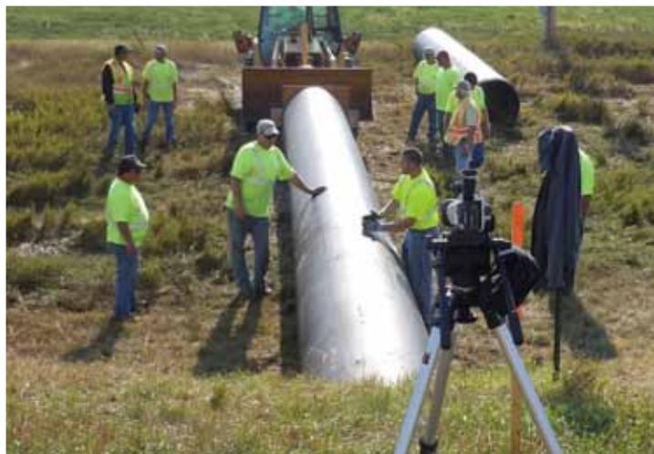
Observers at the demonstration watch the 40-inch Snap-Tite pipe get inserted into the 42-inch CMP.
