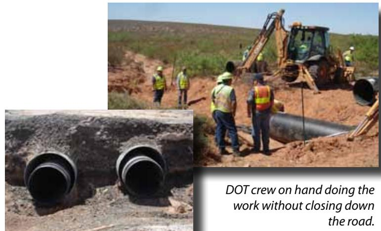
*Two culverts side-by-side with the Snap-Tite liner in place, awaiting grout.*
