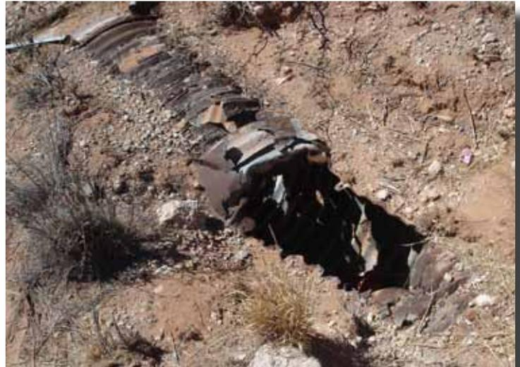
*One of the deteriorated culverts underneath SR 31. This one is severely rusted and eroded on top.*
