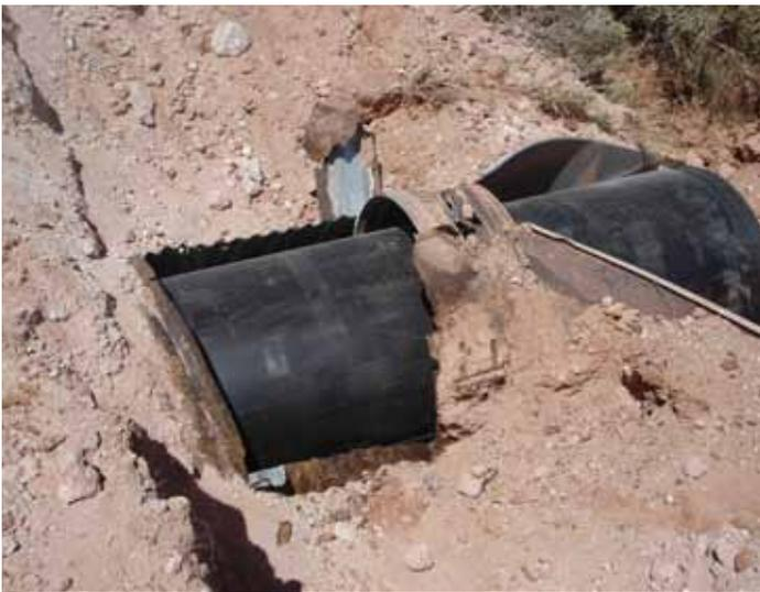
*The Snap-Tite liner lengths are snapped together onsite and slid inside the deteriorated culverts. The Snap-Tite liner is going into another culvert that has disintegrated on top.*
