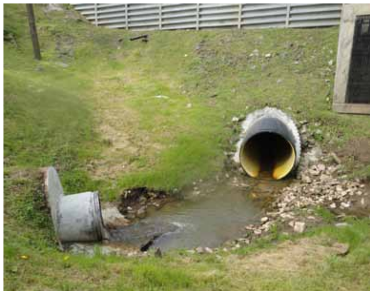
Once the culvert was relined, the flow through the culvert improved.
