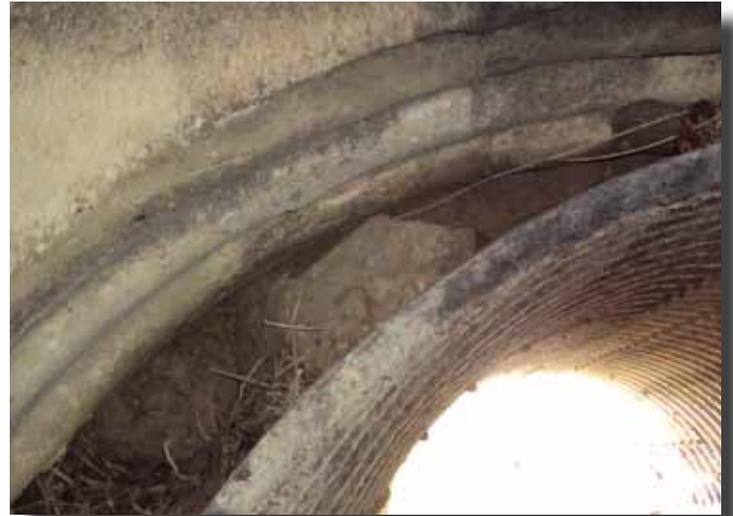
*The old levee culvert was damaged and failing in several areas of the length of the pipe. Flooding was a concern.*
