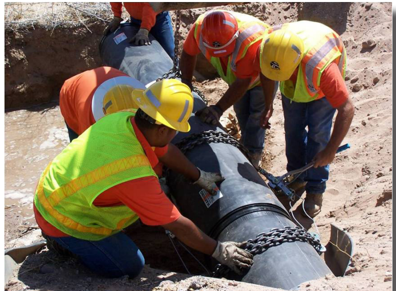
The Snap-Tite pieces mechanically connect with chains & come-a-longs.
