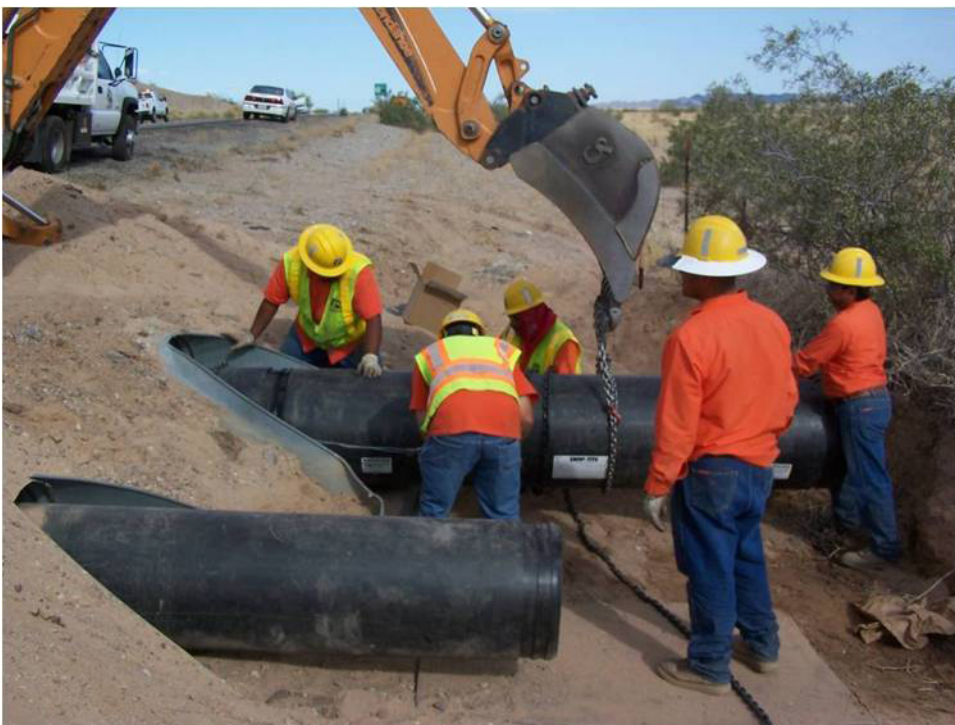
Equipment used to align pipe.
