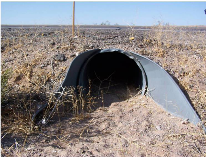
The outside of the culvert to be rehabilitated.
