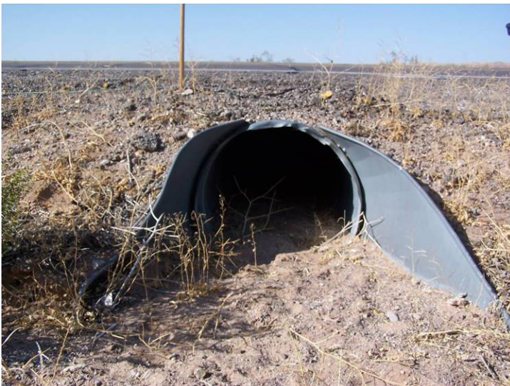
The outside of the culvert to be rehabilitated.
