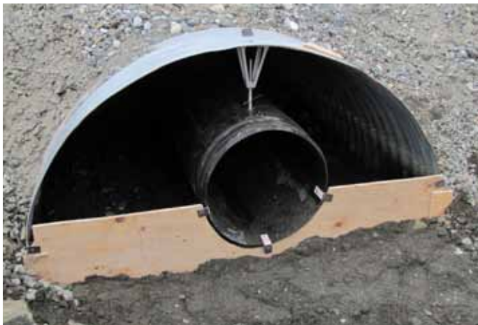
The first bulkhead is created after the pipe liner is inserted and before the grout is pumped in.
