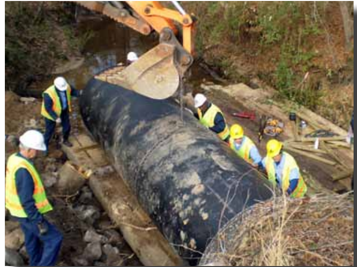
The Snap-Tite® pipe is slid inside the old CMP culvert.
