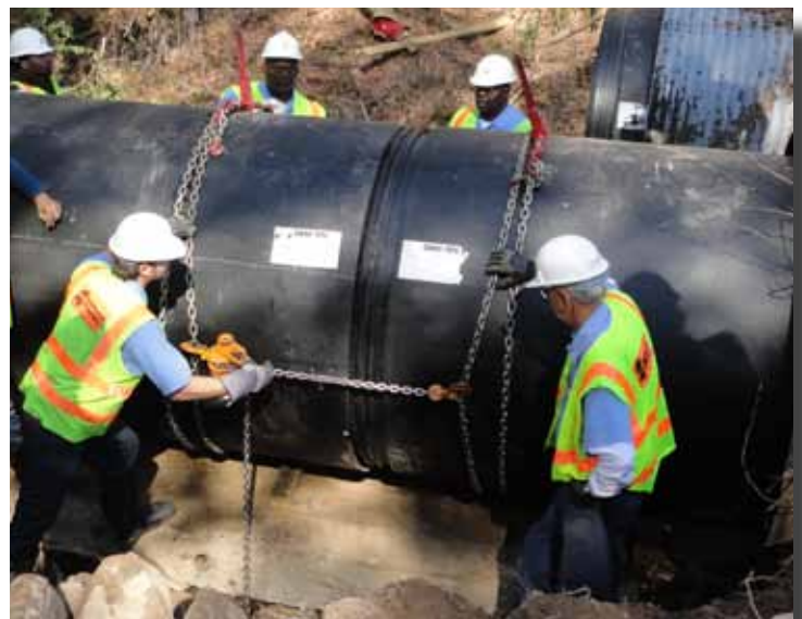
The Snap-Tite® pipe ends are snapped together using only a come-a-long and chains.
