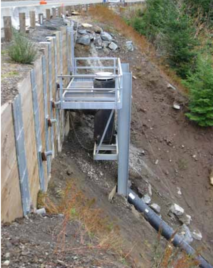
Figure 4: The installation complete.
