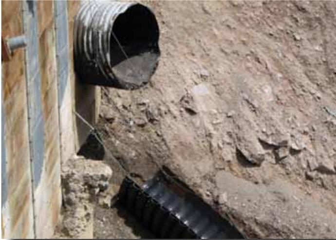
Figure 3: Outfall at the soldier pile wall showing the exposed lagging
