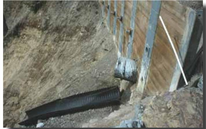
Figure 1: The 36-inch CMP with a half-pipe included as a temporary fix to the failing culvert.
