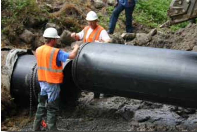
The city of Valdosta crew installs Snap-Tite.
