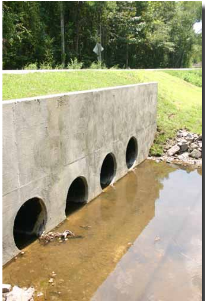
The completely rehabbed culvert.
