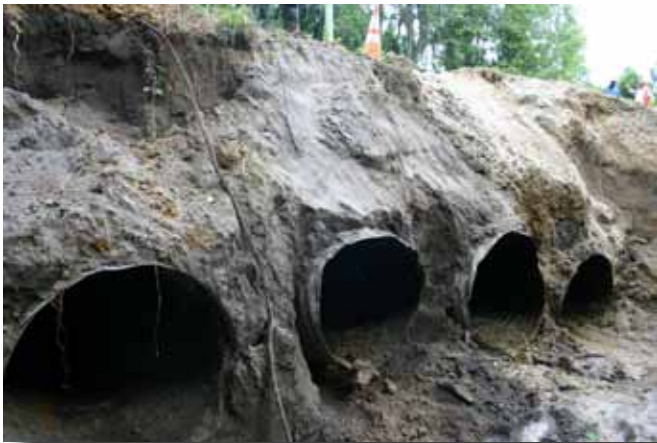
The culvert consisted of four badly corroded pieces of corrugated metal pipe in a row.
