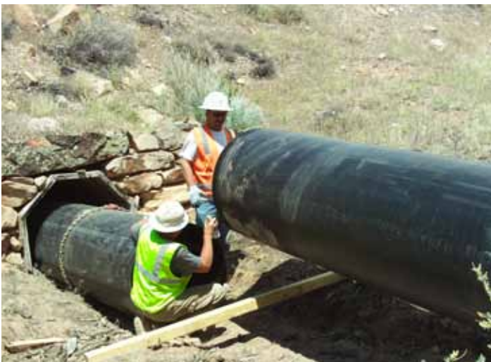
The crew is prepping the 30-inch Snap-Tite pipe for another joining.
