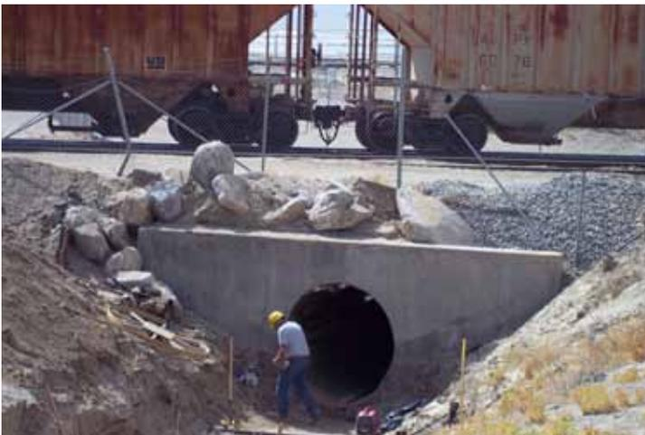
Work takes place on repairing the culvert without disruption to rail service. The Snap-Tite pipe liner and Hydro-Bell are installed under the railway tracks.
