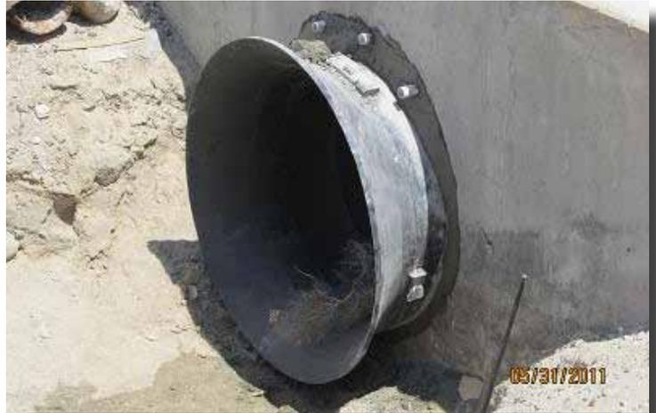
The Snap-Tite pipe with the Hydro-Bell end are in place after installation. The old culvert is relined without any entrance losses.
