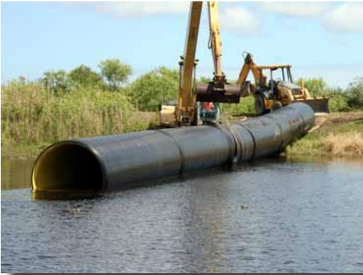
*The electrofused PPT pipe was placed in the water to be submerged under water and pushed into the old pipe.*
