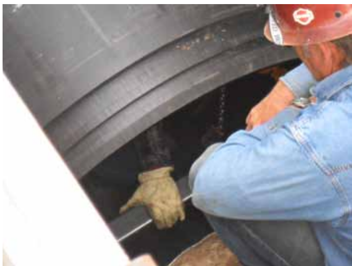
The Snap-Tite® pipe liner ends are snapped on the inside of the pit and then pushed through the old pipe to reline it.
