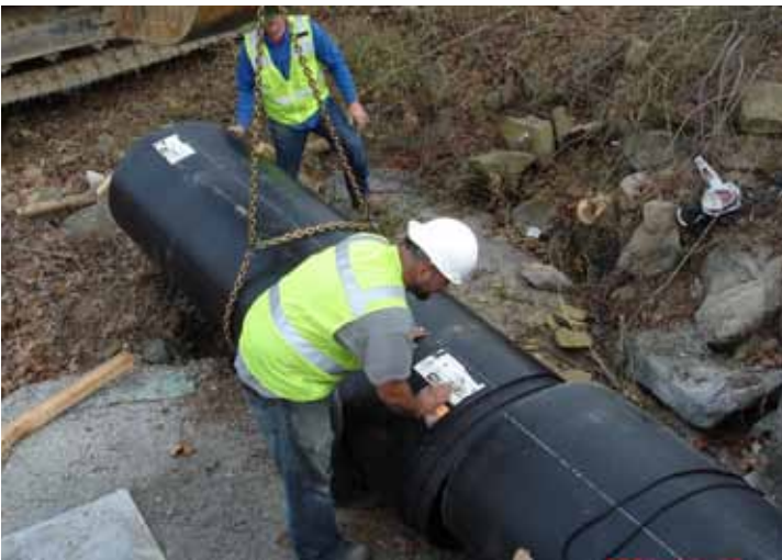
The machined Snap-Tite male end is about to be 'snapped' to the female end of the pipe.
