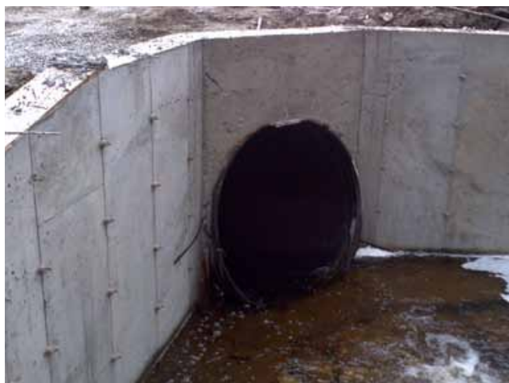
The fully lined pipe outperforms the pipe it replaces and flow is maximized.
