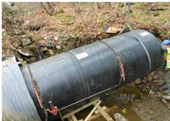
The snapped sections of pipe are slid inside the old CMP, completely lining the deteriorated pipe.
