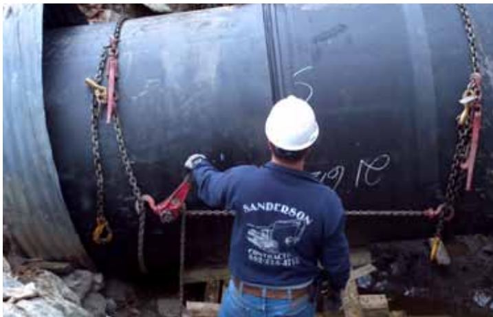
Sections of the Snap-Tite pipe are snapped together using only a come-along and chains.
