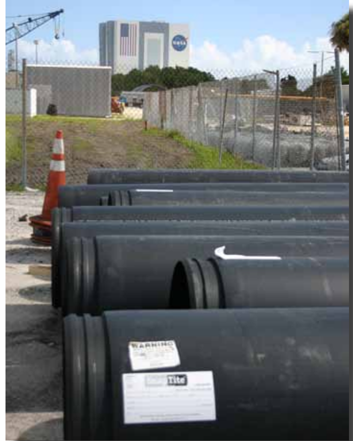
Snap-Tite is delivered to the Kennedy Space Center and awaiting installation.
