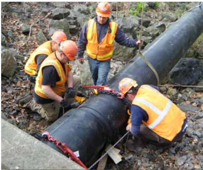
After the Snap-Tite pipe male and female end are snapped together, the joined section is slid inside the old CMP.
