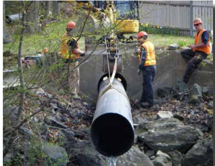
*Snap-Tite pipe is slid inside the old storm drain. Relining the pipe is quicker and safer than a dig and replace method.*
