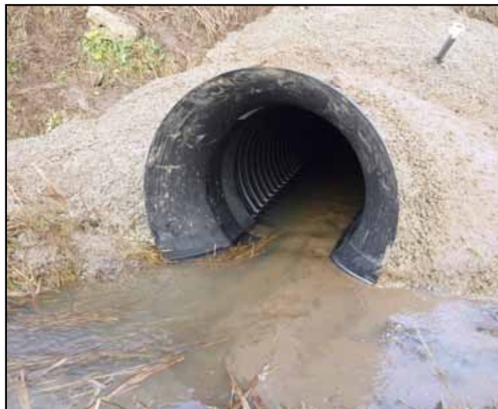
A view of the upstream side of the IOP pipe with the Hydro-Bell attached, after the project is completed.
