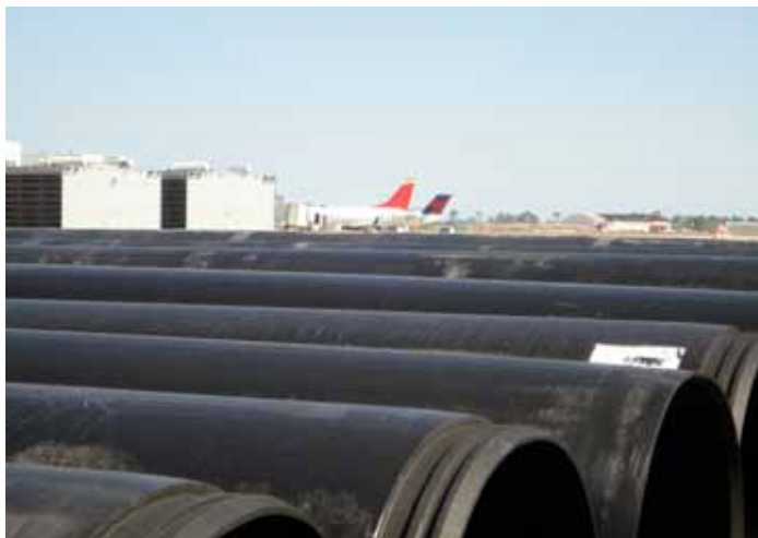
Snap-Tite supplied 49-foot sections of 42-inch and 48-inch diameter HDPE Snap-Tite pipe. The pipe is pictured here awaiting installation.
