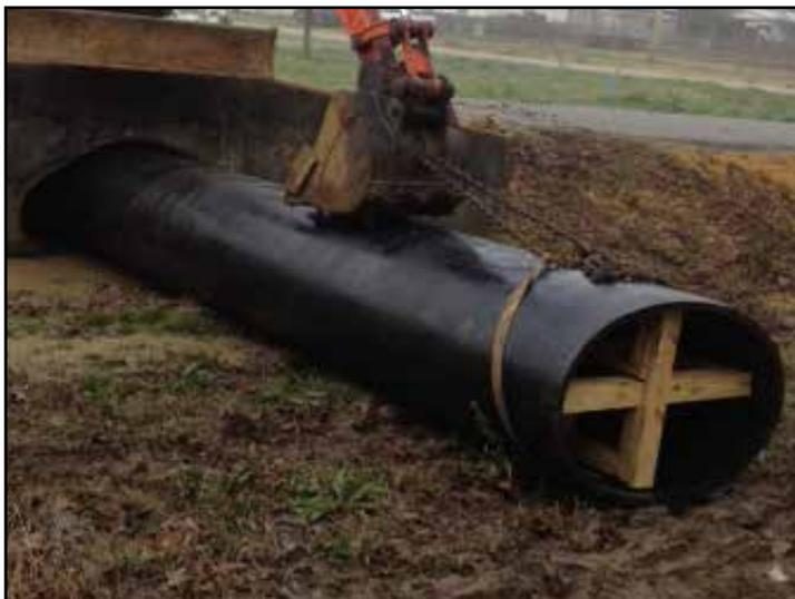
*Snap-Tite pipe liner is pulled inside one of the old culverts.*
