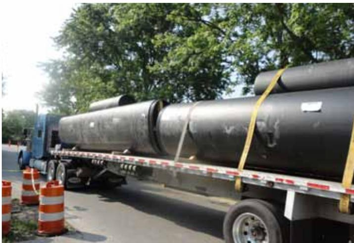
*Snap-Tite supplied sections of ovalled Snap-Tite HDPE pipe to line the oval culvert. Snap-Tite delivered a total of 190 feet of pipe.*
