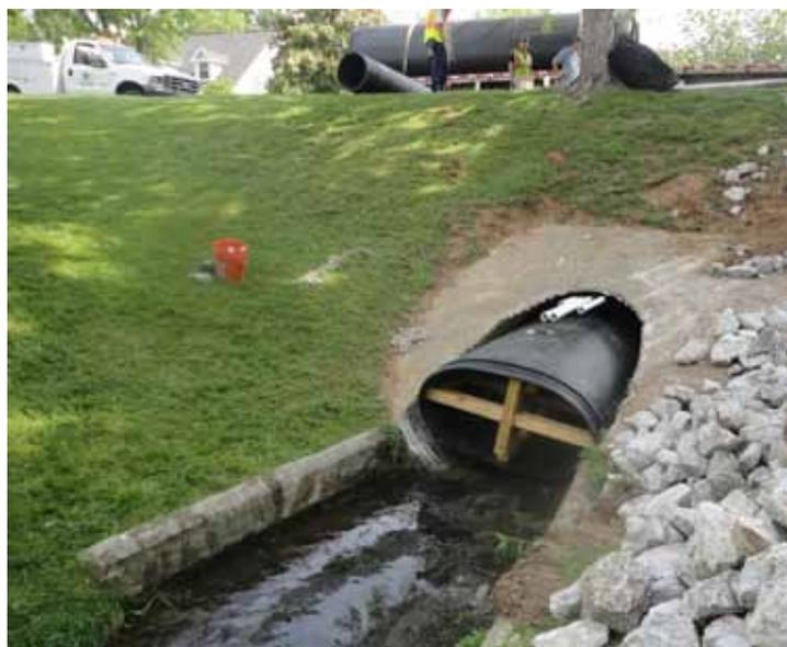
The Snap-Tite pipe liner was slip-lined into the old culvert one section at a time. Each section was snapped together using a come-a-long and chains.
