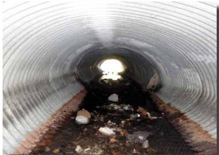
*The original culvert was corroded and in bad shape. It was located in a residential neighborhood so if it failed it could compromise the foundation of some homes.*
