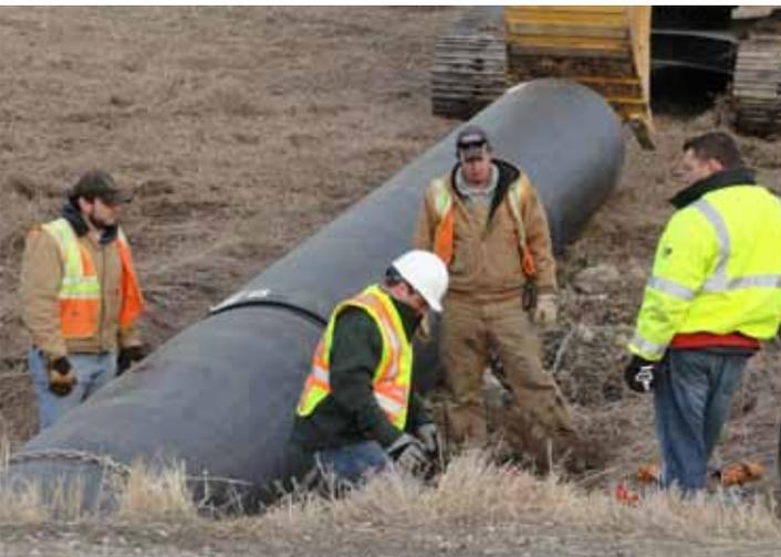
*One section of the liner is first inserted into the CMP and then snapped to another section.*
