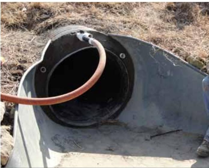
*Grout is pumped in to fill in any voids in the annular space between the liner and CMP.*
