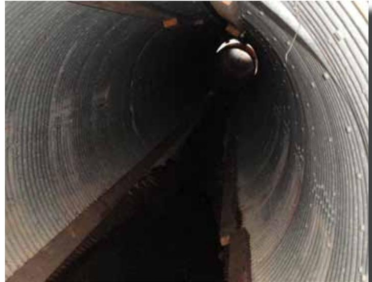
*Inside the old CMP culvert, showing signs of wear and deflection.*
