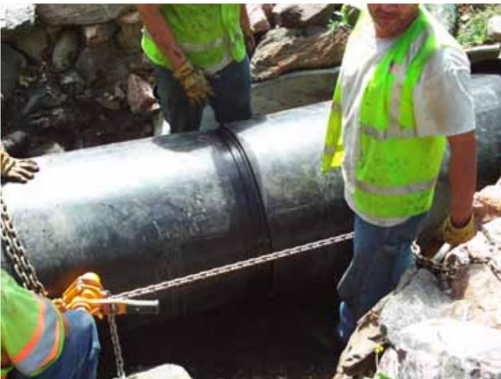
*SEMSWA crews join the Snap-Tite pipe sections using a come-along and chains.*
