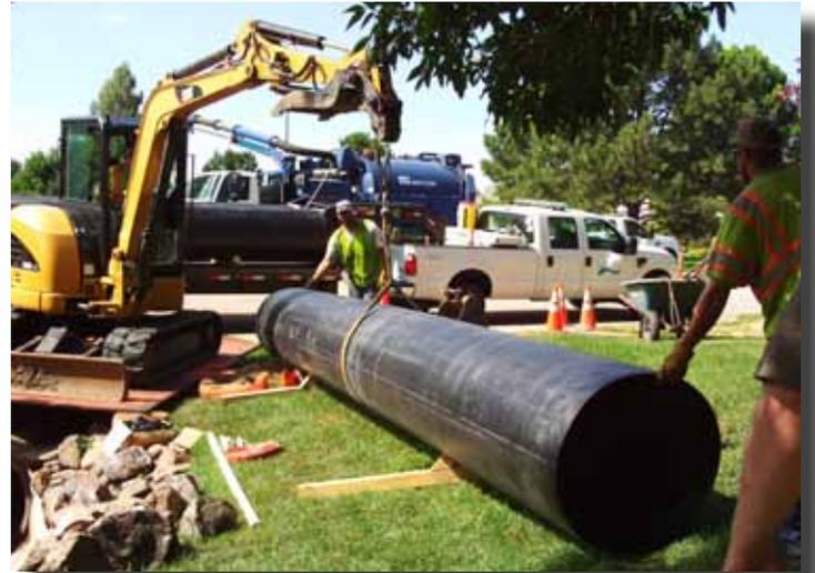
*The Snap-Tite pipe is moved in place to line the old CMP using a mini excavator.*
