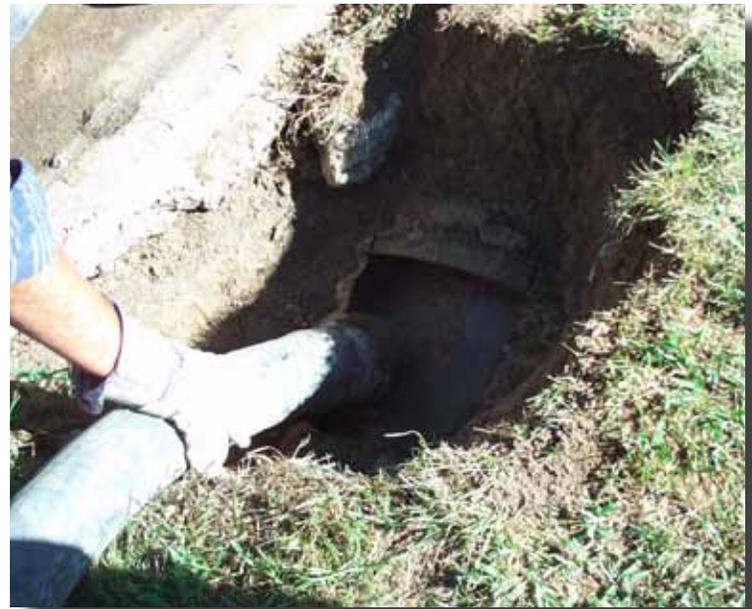
*Any annular space between the old CMP and the Snap-Tite pipe liner is filled in with grout.*
