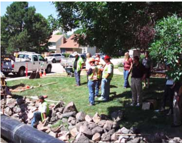
Demonstration attendees view the first installation of the Snap-Tite pipe liner.
