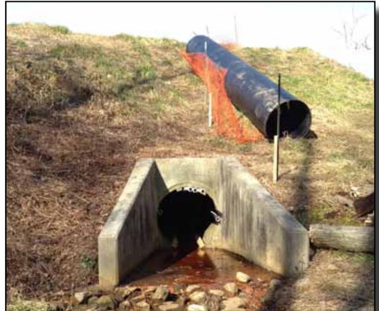
*Snap-Tite pipe will be slid inside the old culvert during the installation process.*
