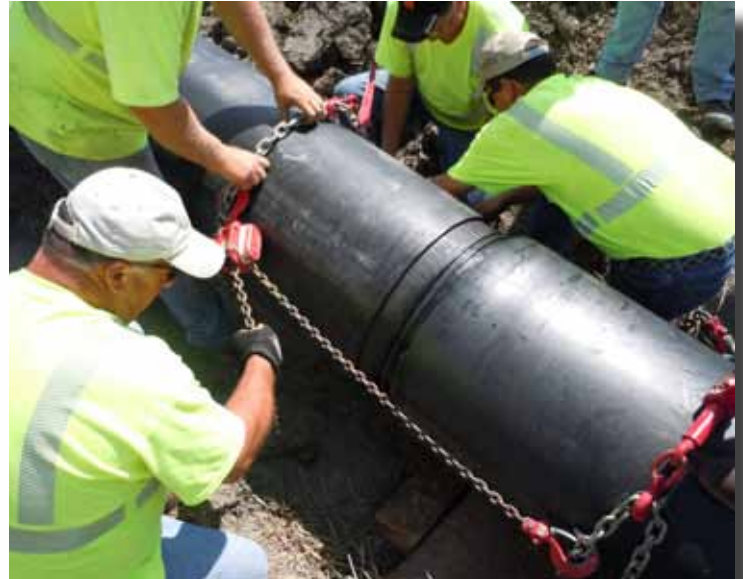
The machined Snap-Tite ends are joined together using only come-a-longs and chains.
