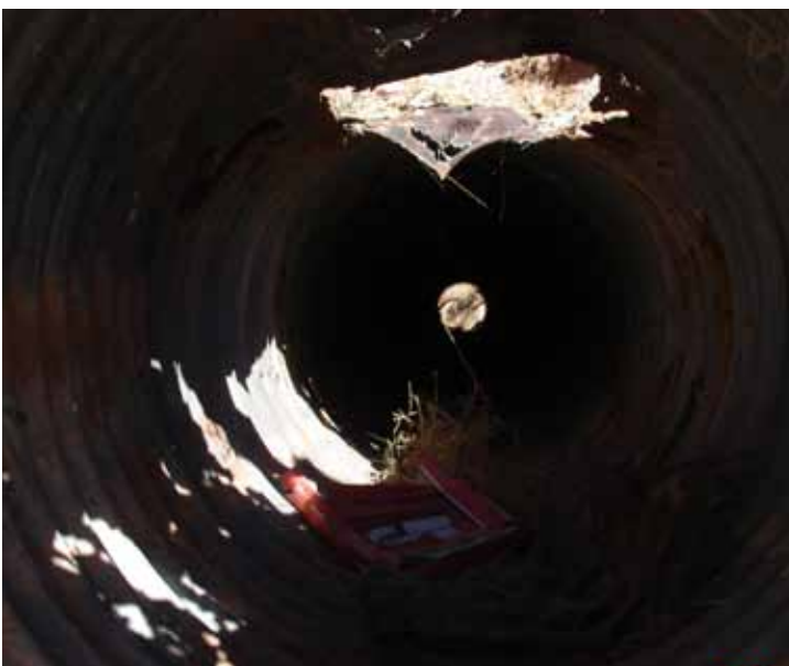
A view of the culvert from the inside. Note the hole at the top where the culvert has completely deteriorated and caved in on itself.
