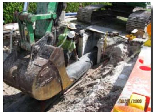
*Snap-Tite pipe pushed in the culvert.*
