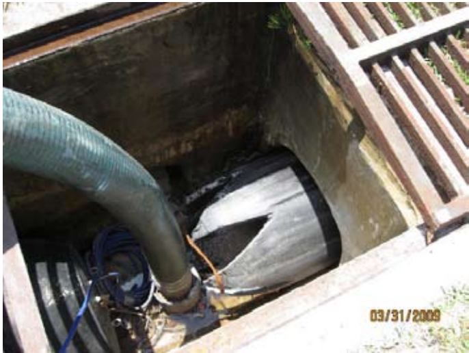
The nose cone coming through the culvert.
