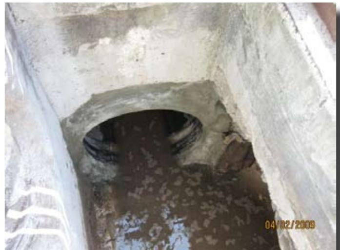
*The rehabilitated culvert, with water flowing through.*
