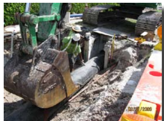
Snap-Tite pipe pushed in the culvert.
