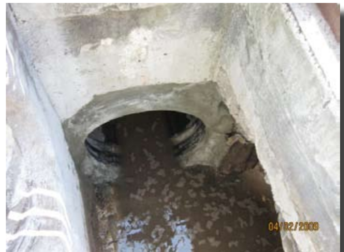
The rehabilitated culvert, with water flowing through.
