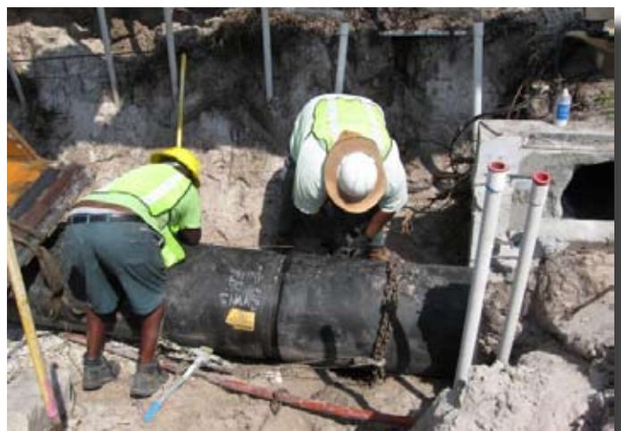
*The pipe "snapping" together.*
