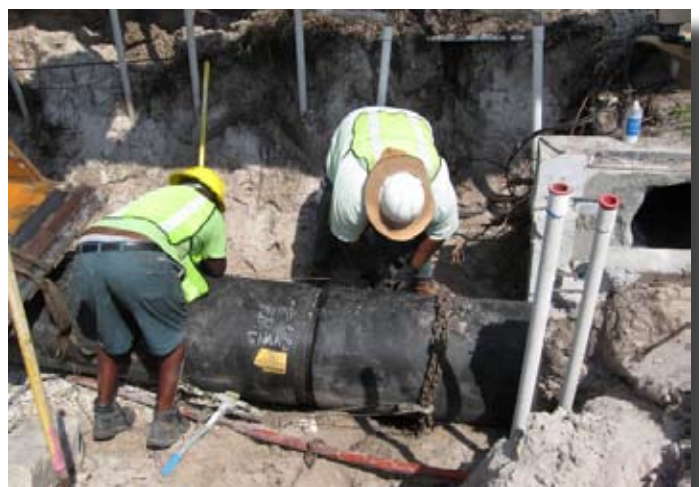
The pipe "snapping" together.
