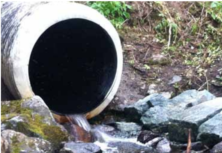
Culvert relined with Snap-Tite pipe.
