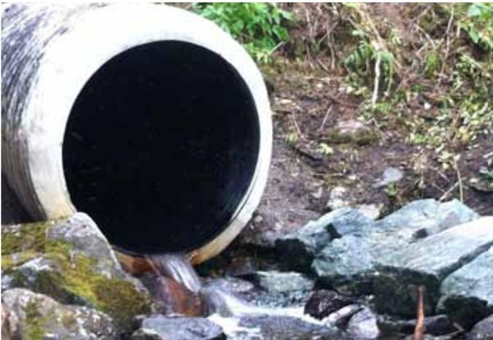
*Culvert relined with Snap-Tite pipe.*
