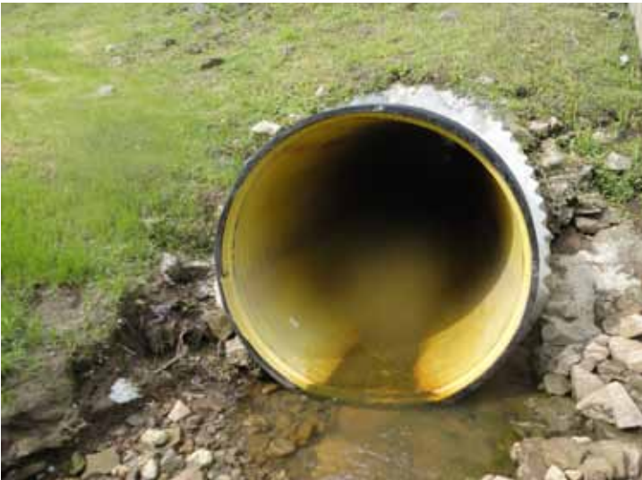
Once the culvert was relined, the flow through the culvert improved.
