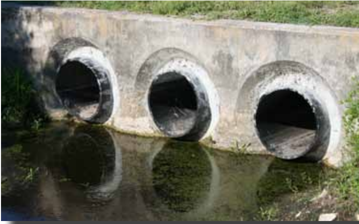
The three culverts after they are relined with Snap-Tite.
